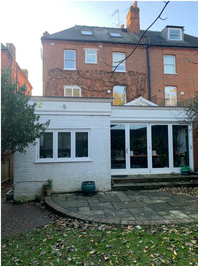
Fig. 3 Rear (north elevation) with its ground floor rear extension.
