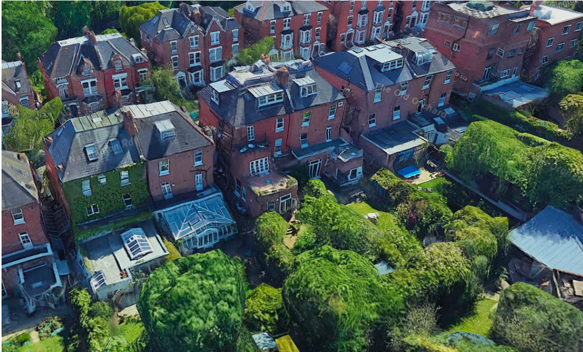
Fig.10 The context of 16 Nassington Road: all five houses to its west have dormers
