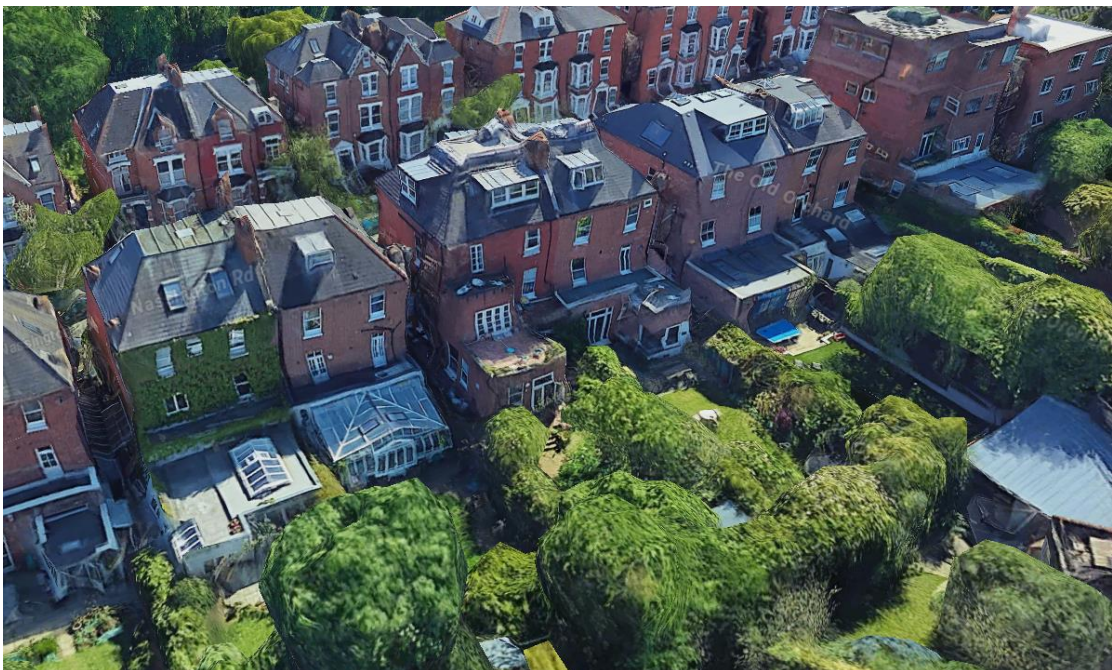
REAR DORMERS AT 6-14 NASSINGTON RD
