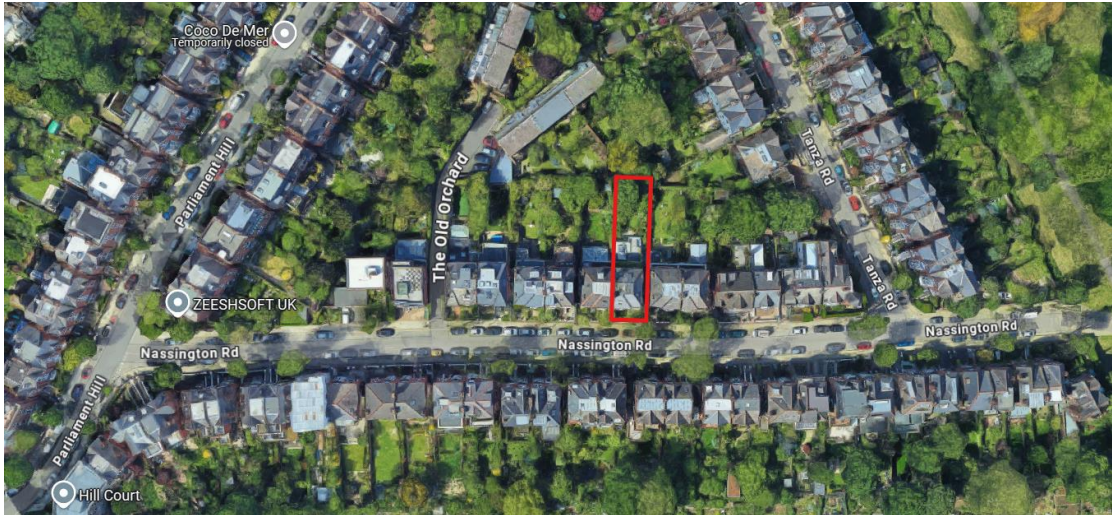
AERIAL VIEW OF SITE
