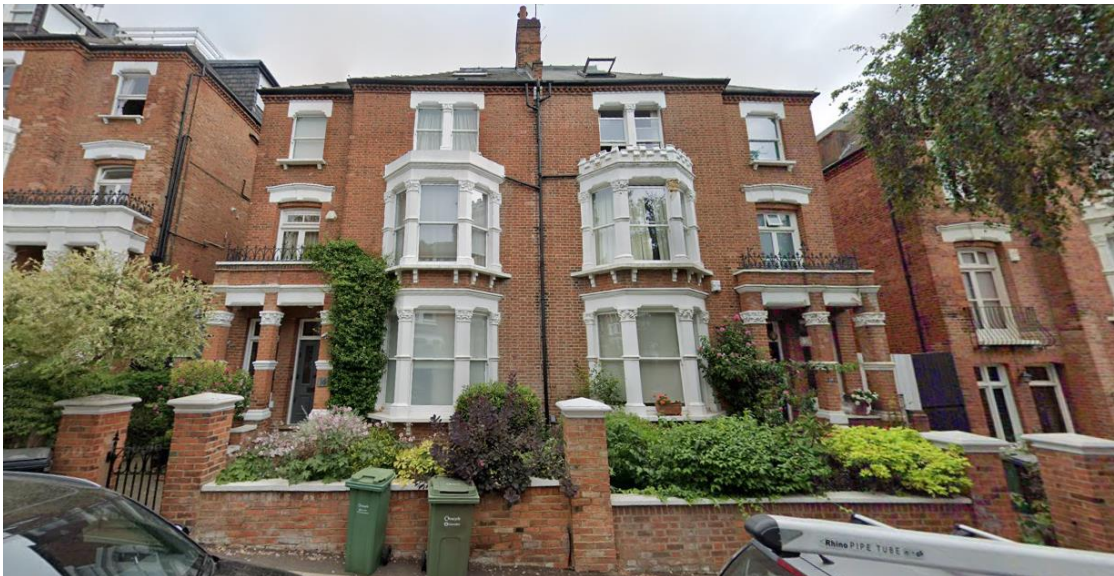
VIEW FROM STREET LEVEL OF 14 & 16 NASSINGTON ROAD
