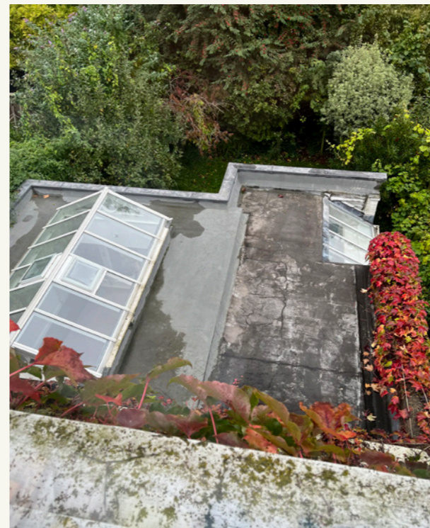
3. View of roof of existing extensions
