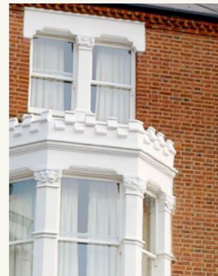
Existing red brick and stucco
