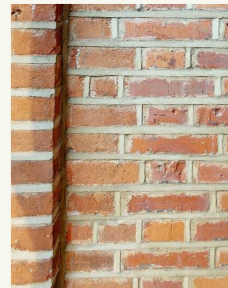
Existing red brick
