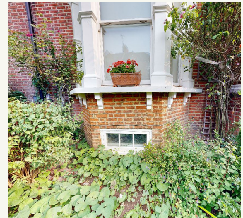
4. View of front window to basement
