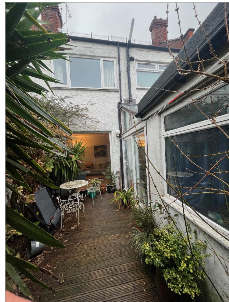
PHOTOGRAPH OF REAR ELEVATION TAKEN FROM REAR YARD
