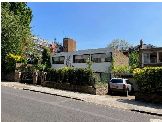
Fig.3 view from street showing 63 Ornan Road
