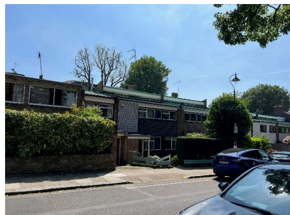
Fig.4 view from street showing 59 Ornan Road
