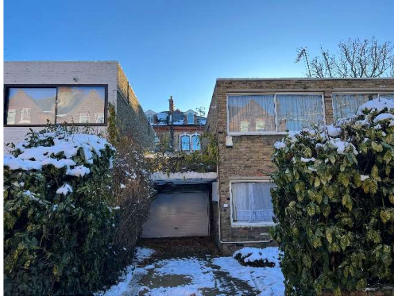
Fig.5 view from street showing 63 & 61 Ornan Road
