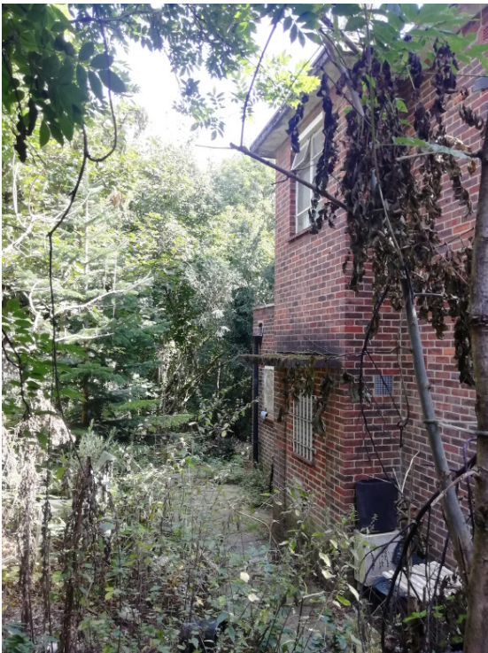
3. Existing front entrance (now blocked up)
