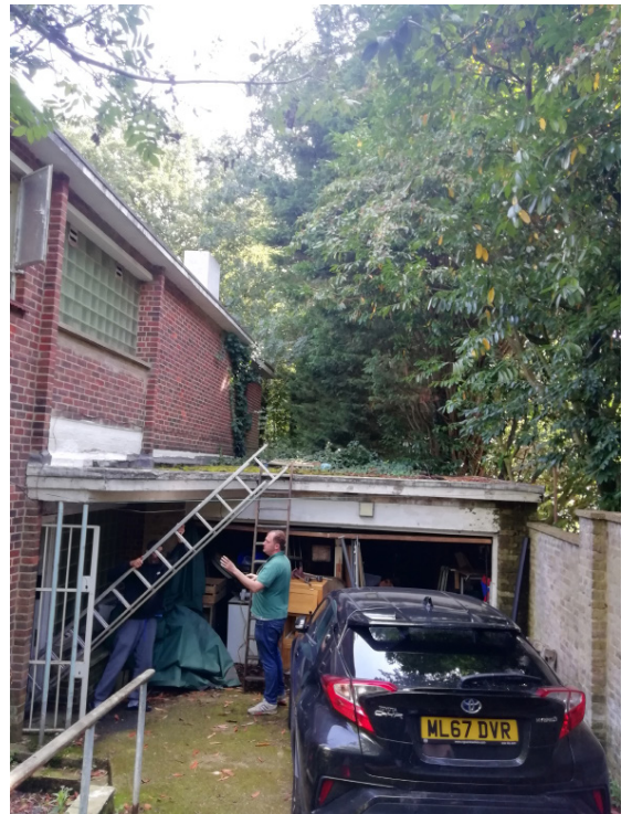
4. Existing double garage and side entrance
