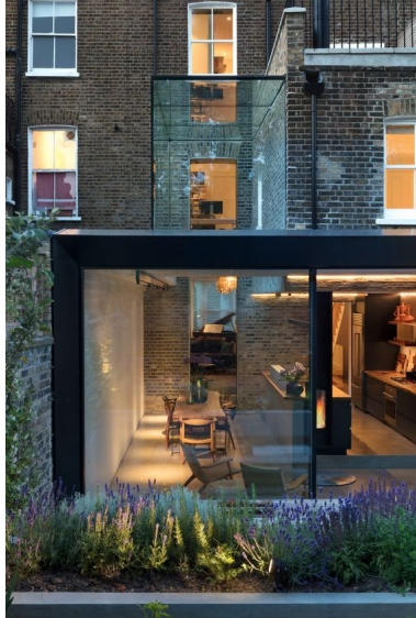
Rear extension with glass box rooflight
