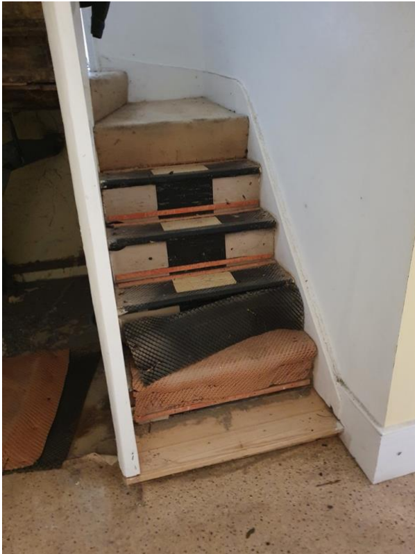
Figure 1: Existing stairs at lower ground floor level
