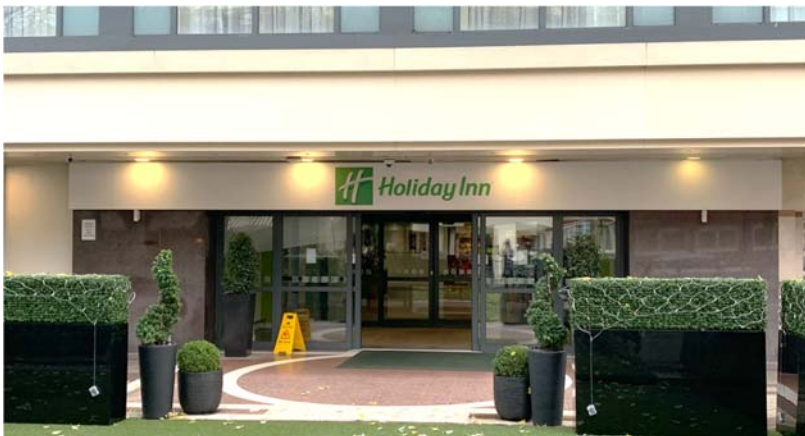
Photo 05 looking south at the main hotel entrance which is adjacent to the bar entrance. Note the use of metal frame for the doors and the windows, and polished stone cladding.
