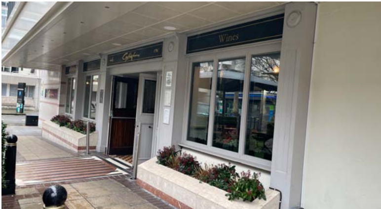
Photo 02, the same area. Existing bar entrance doors, planter, and windows. Timber, paint finish. The planter is in polished stone. The doors have no lower vision panel, contrary to current wheelchair access requirements.
