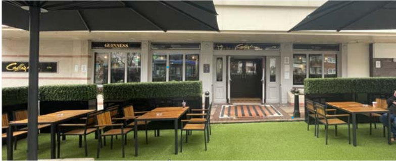
Photo 01. Looking south. Showing the existing bar entrance doors (outer pair of the lobby are open) and structure, dressed in timber. Paint finish. Polished stone cladding elsewhere. Decorative tiles to the entrance area. Area in front set out with astroturf and seating, for compliance with public area smoking. Signage above the doors and windows.
