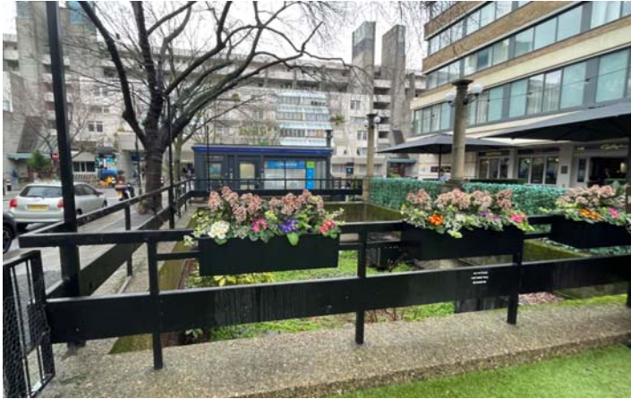
Photo 04, looking east, of the sunken garden area. Metal guarding painted black. The metal box structure in the background is the access point for the basement gym. This structure is also metal framed.
