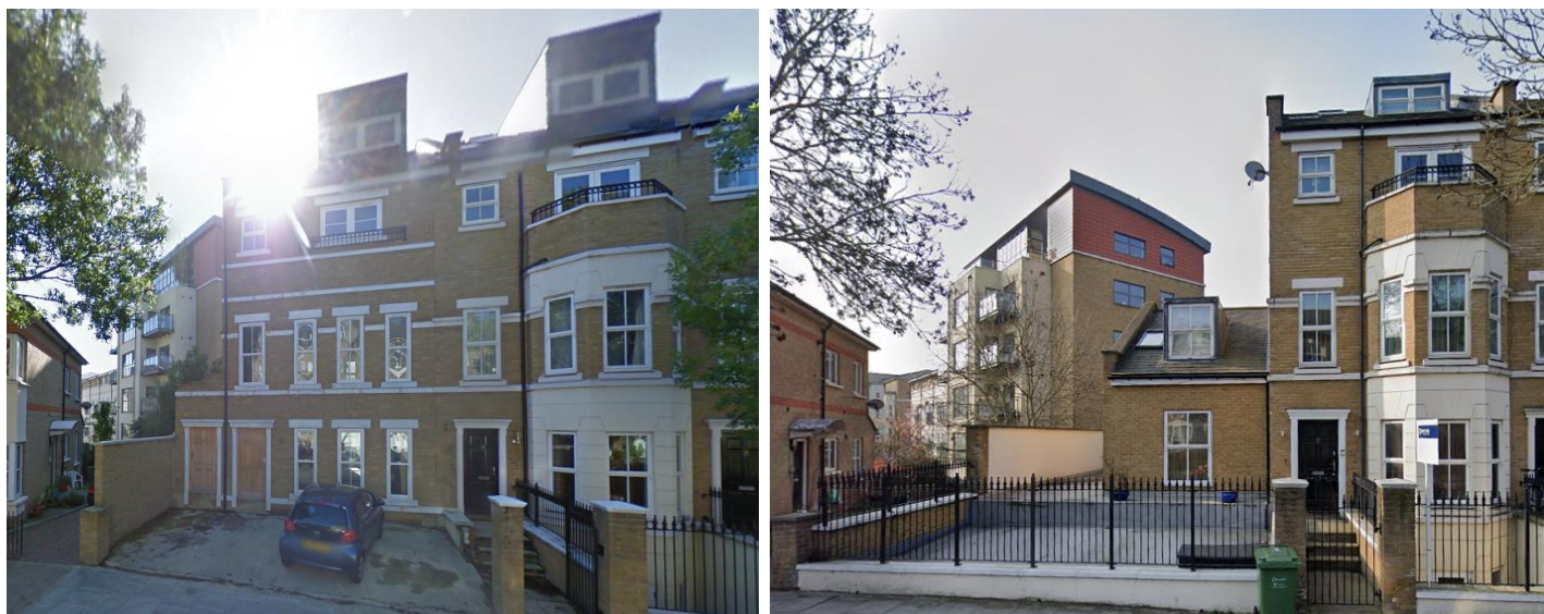
Figure 1. Front elevation of 20 Busby Place before (left) and (after) enforcement action concerning the unlawful four-storey, basement, and sub-basement construction.
