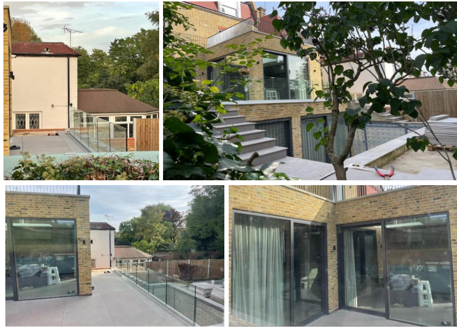
Photograph 21,22,23,24 : Unit at 251 - Rear elevation
