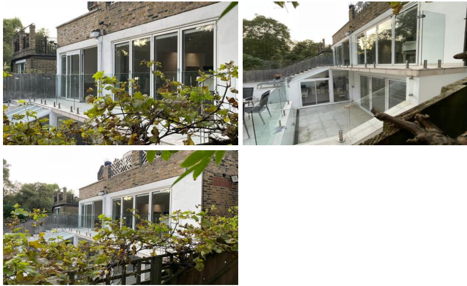
Photograph 18,19,20 : Unit at 255 - Rear elevation
