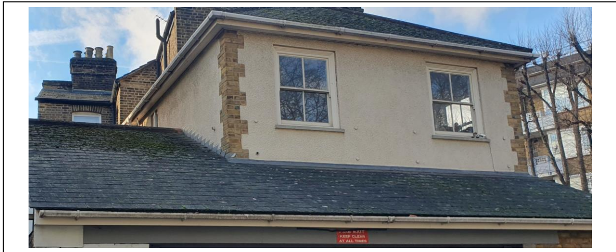
Figure 3: Site Location Measurement Pictures
