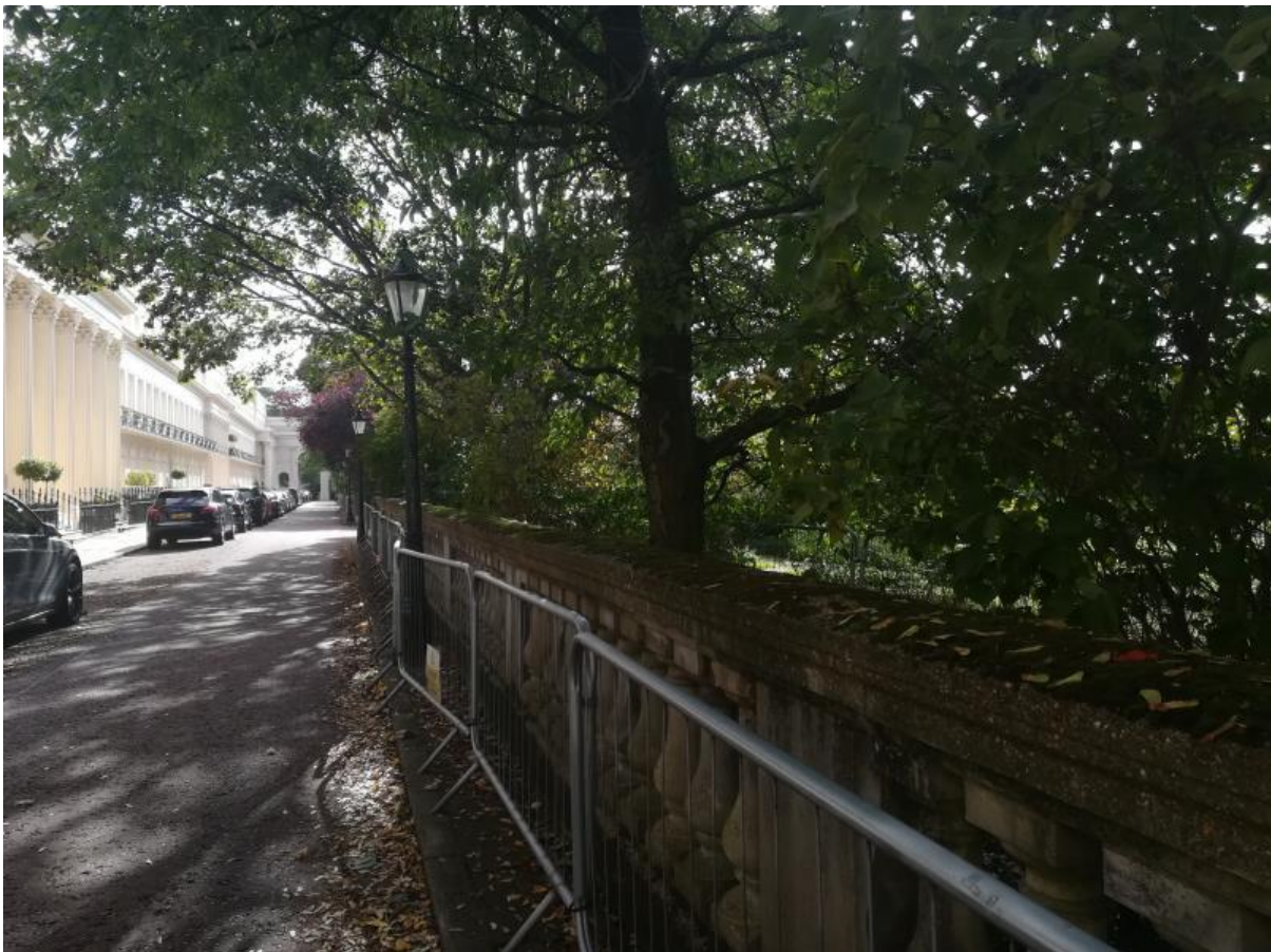
Figure 11: Looking south along the higher side of the retaining wall from the public highway of Chester Terrace, showing the clearance of T223 (front centre-right) as a general point of reference.
