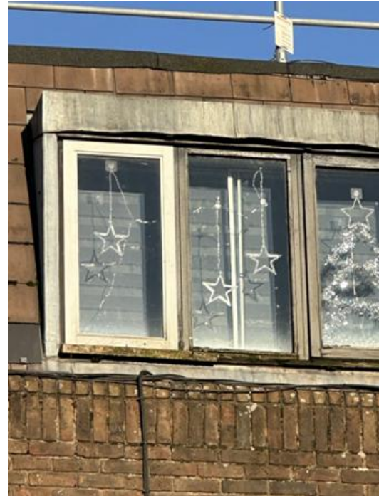
Windows to Third Floor (In Mansard)
