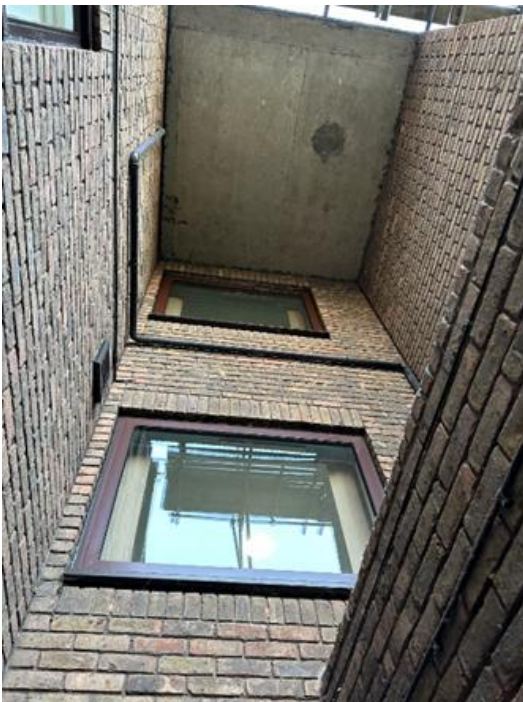
Windows to First and Second Floors
