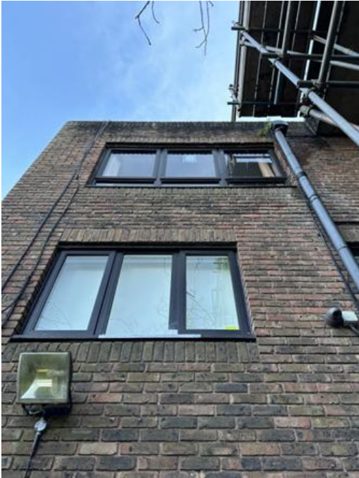
Windows including W03 to First/Second Floors
