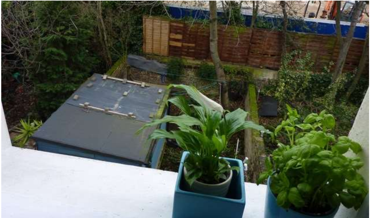
27 Oval Road rear with Party Wall with 29 Oval Road
