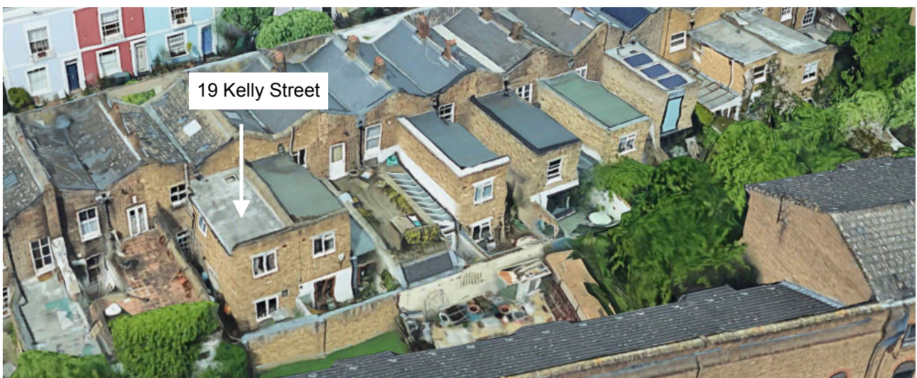
Fig.02 – bird's eye view of 19 Kelly Street (highlighted) in relation to its immediate context. It can be noted that other neighbouring and nearby properties have undergone extensive development in the form of infill extensions and roof terraces.
