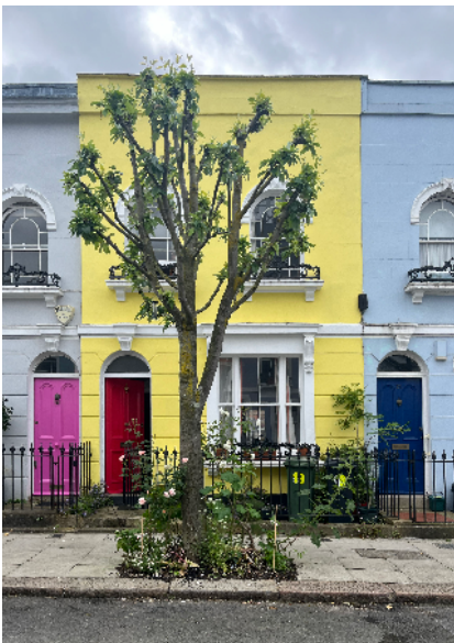
Fig.03 & 04 (left and middle) – Existing front elevation with mid C19. stucco with rusticated ground floor, round-arched doorway with panelled door and fanlight moulded bands, cornices and console brackets, wide bracketed sills with elaborate cast-iron guards, sash windows. Fig.05 (right) – decorative corbels in the hallways to be retained
