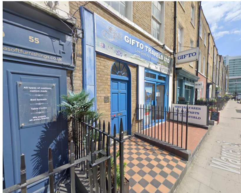
Figure 6 Existing shopfront at No.56 Warren Street (Source: Google Street View)
