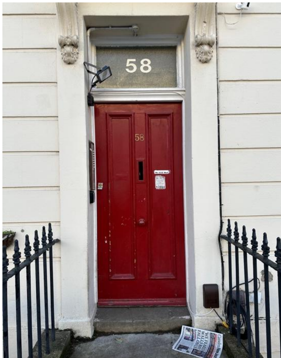
Existing Front Entrance Door
