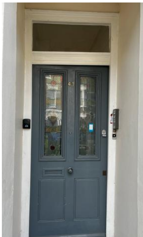
Front Entrance Door
