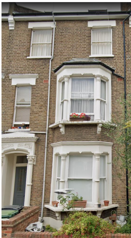
The Site viewed from Roderick Road.
