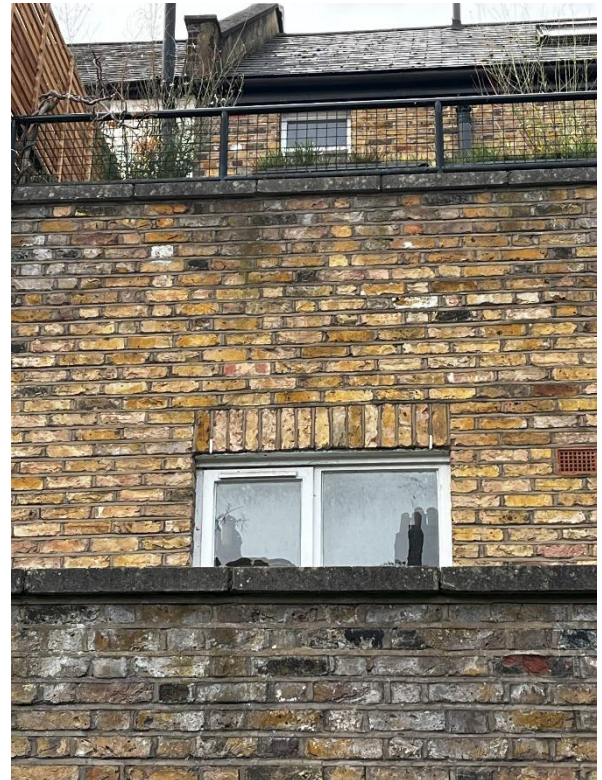
Upper Floors Rear Windows
