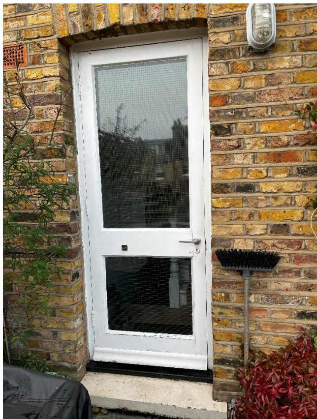
Rear Exit Door to Garden
