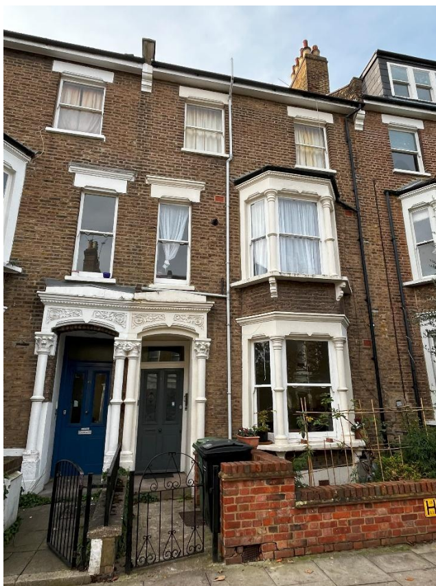
The Site viewed from Roderick Road.
