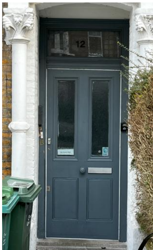
Front Entrance Door
