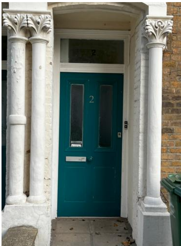
Front Entrance Door
