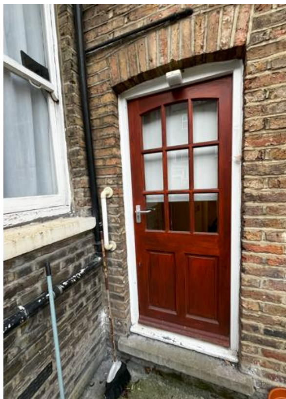
Rear Exist Door
