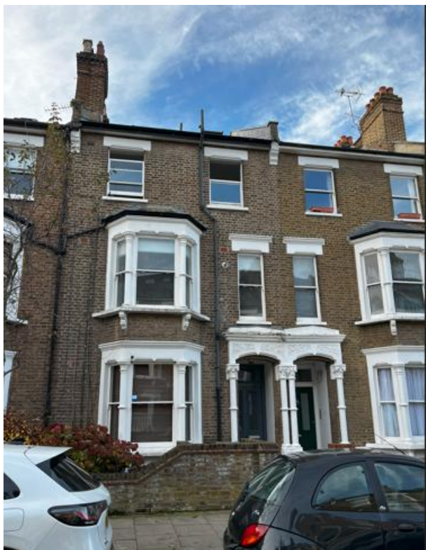
The Site viewed from Roderick Road.
