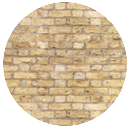
Existing brickwork facade at first floor
