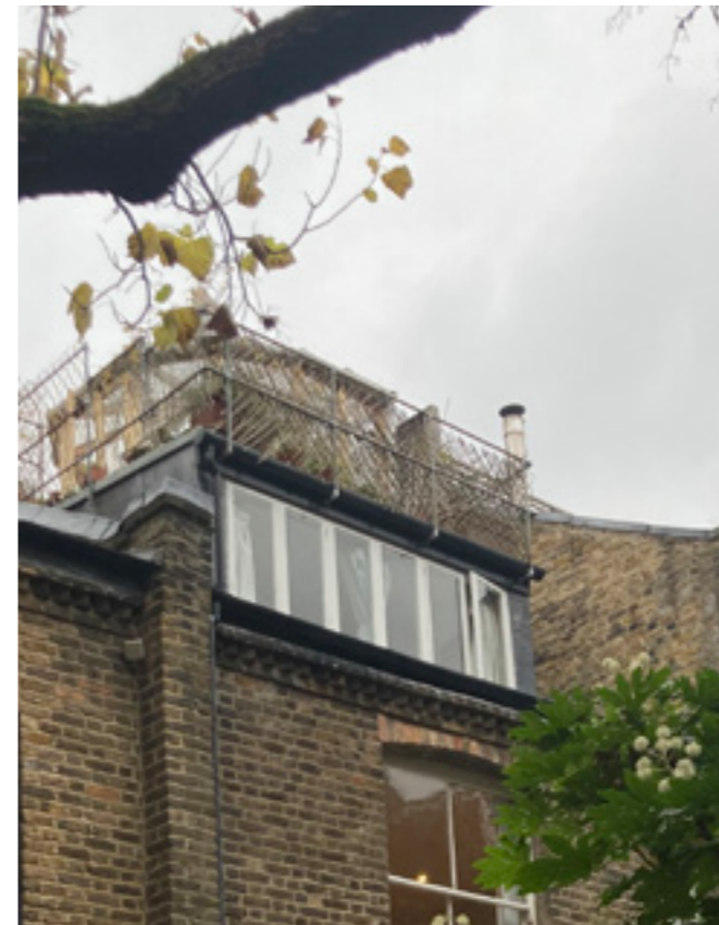
Dormer (added in 1970s) housing master bedroom
