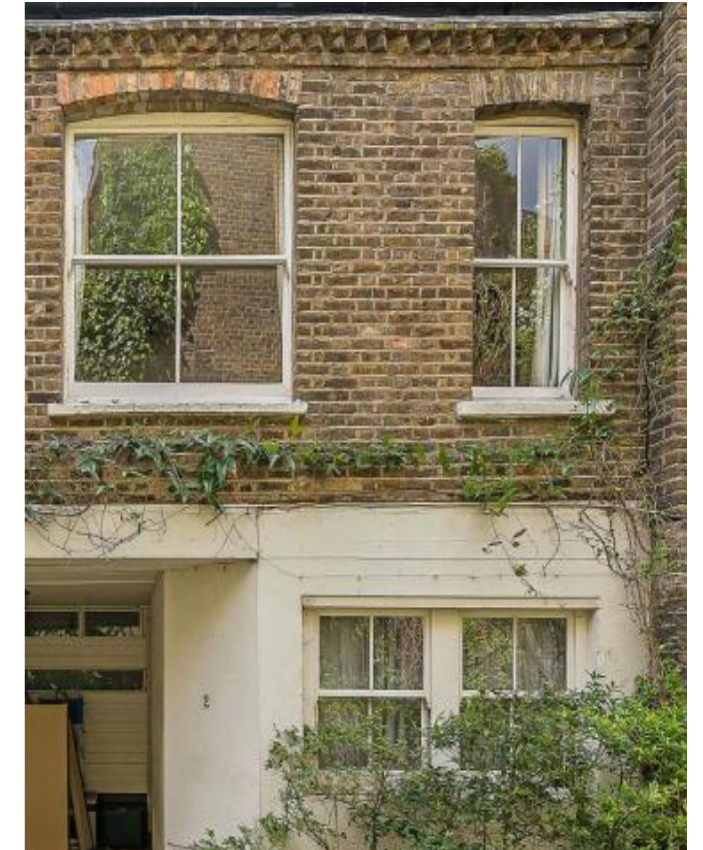
Timber sash windows
