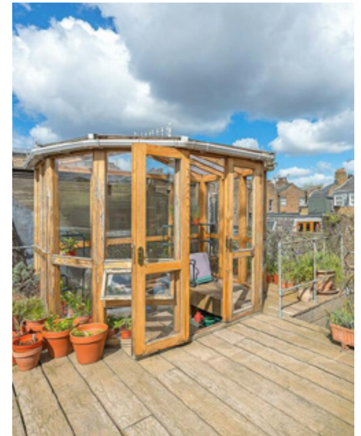
Single-glazed timber conservatory sitting on roof deck structure
