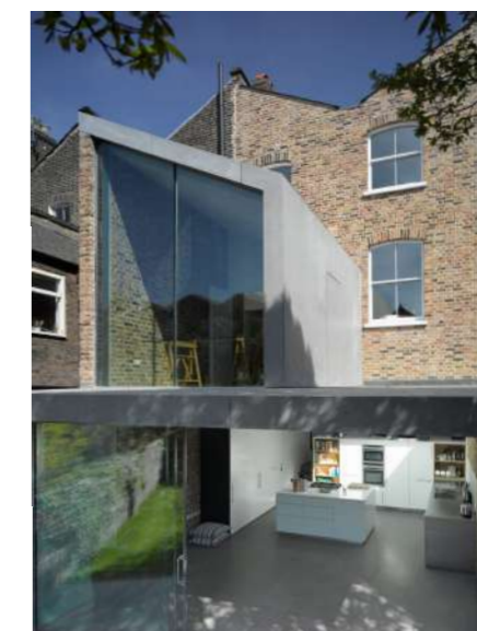
Fig.8 Artificial slate used at the rear of an RDA project in Kentish Town
