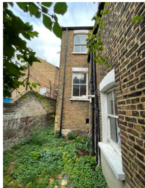
Fig.4 Area of residual space between rear closet and boundary wall
