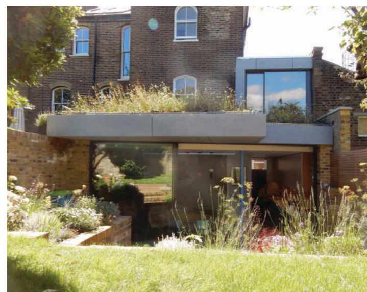
Fig.7 Artificial slate fascia used at the rear of 93 Chetwynd Road
