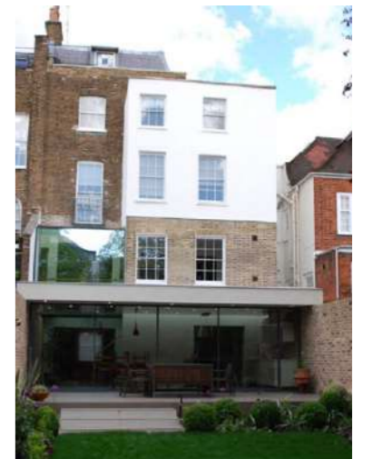
Hamilton Terrace, NW8 - Extension & modernisation of grade II listed terrace house.
