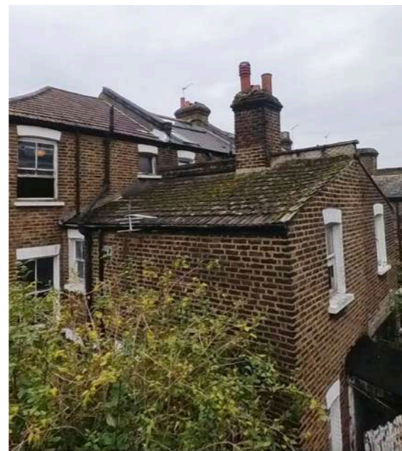
Fig.5 Photo of cement tiles on both roofs
