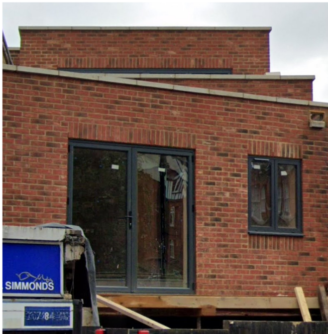
Photo of the front façade of the as-built building
