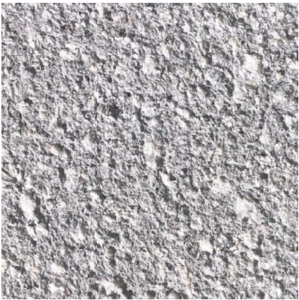
8 Proposed Exposed Aggregate Concrete Finish to Internal Face of Parapet
