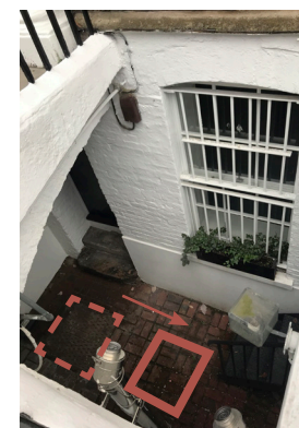
a. Existing manhole to front lightwell shifted out
