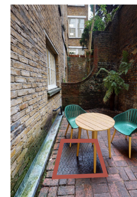
b. Existing manhole to rear courtyard shifted out
