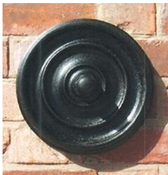
Fig (ii) – proposed bulls eye pattress plate (size 20.3cm diameter)
