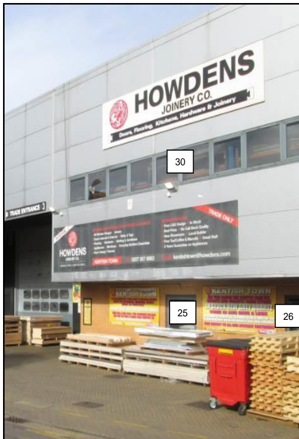
Unit B and Unit 2000 Regis Road
