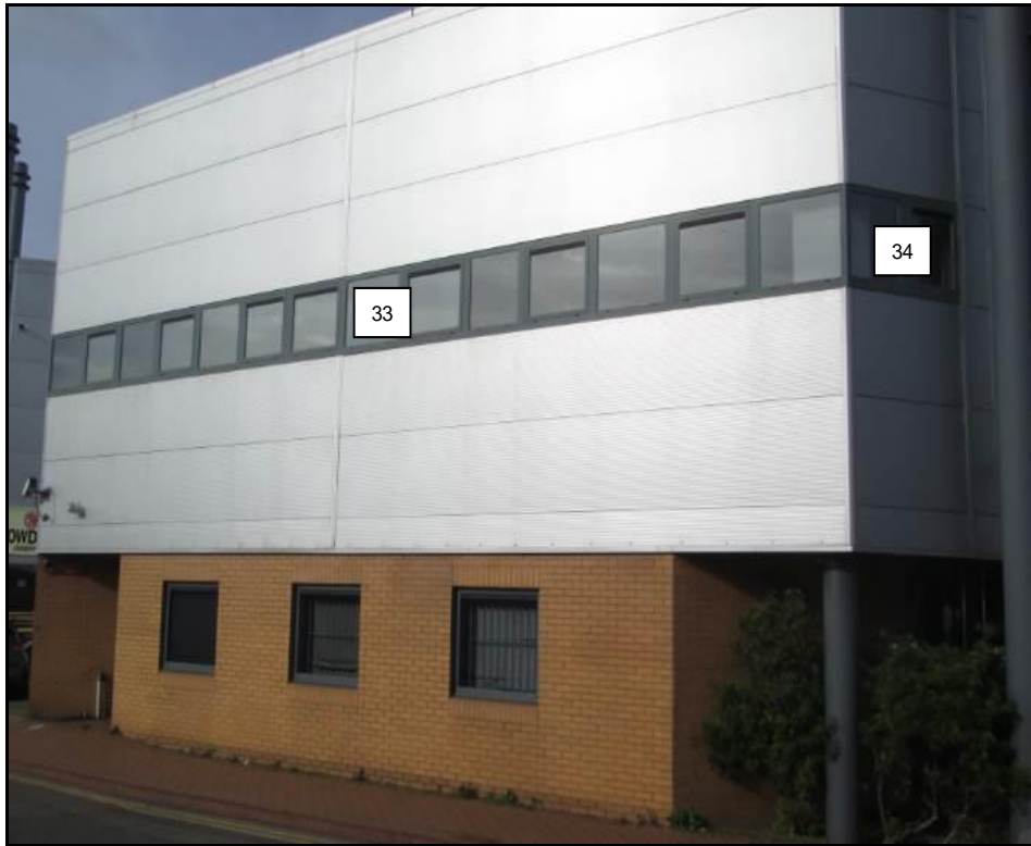
Unit B and Unit 2000 Regis Road
