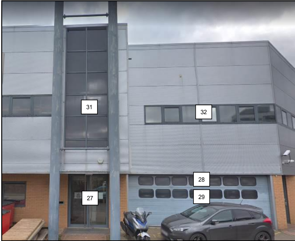
Unit B and Unit 2000 Regis Road
