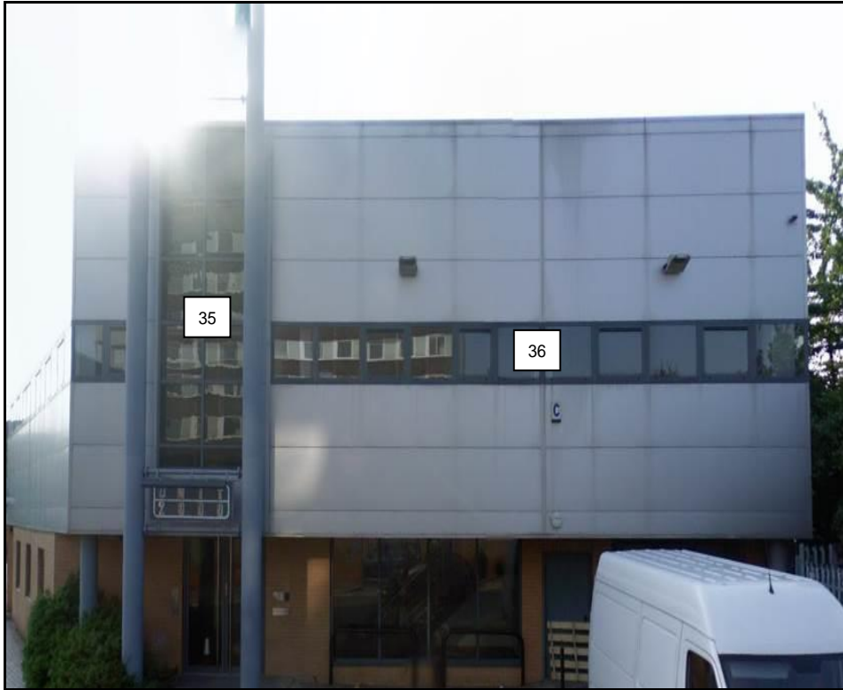
Unit B and Unit 2000 Regis Road
