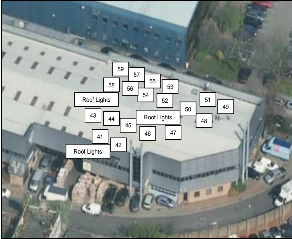
Unit B and Unit 2000 Regis Road
