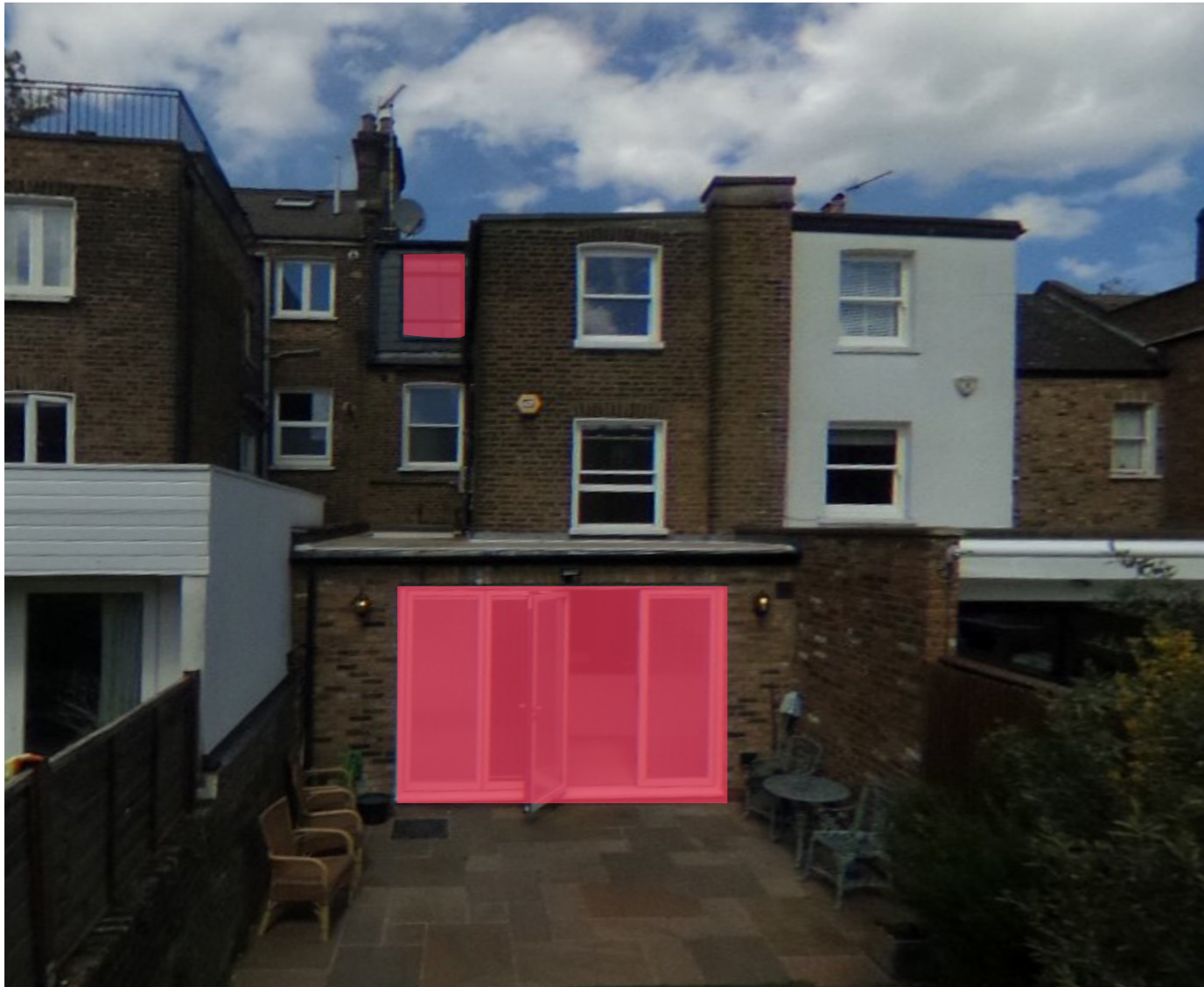
Existing rear view
