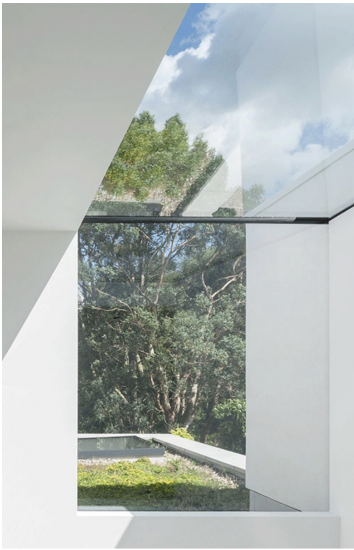
eaves rooflight in side return
