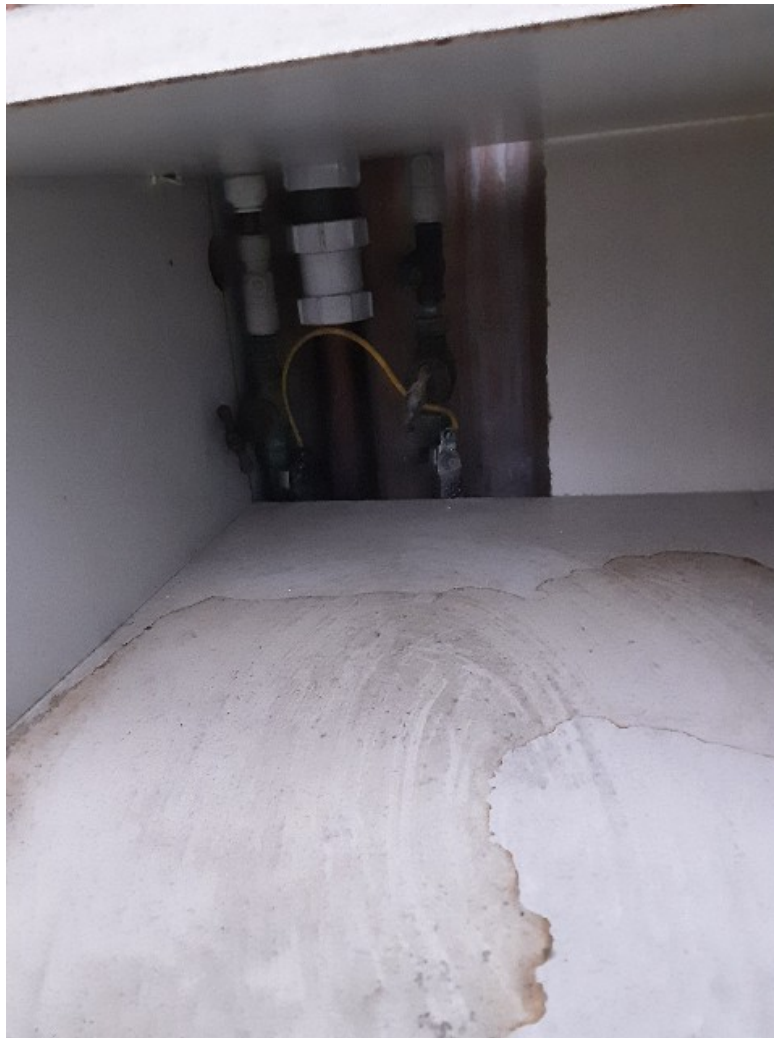
Photo Earth Bonding 1
