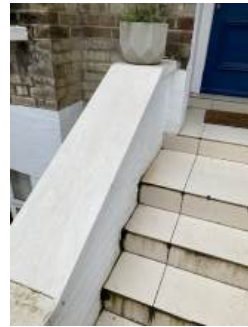
Existing tiled treads risers & painted cappings
