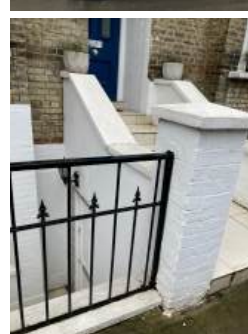
Existing railings tiled treads & risers & painted cappings
