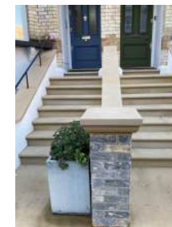
York stone steps and cappings at numbers 11 & 12
