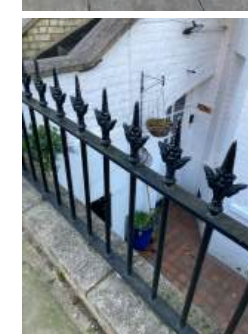
Example of proposed Finial to railings very commonly found on Gayton Road
