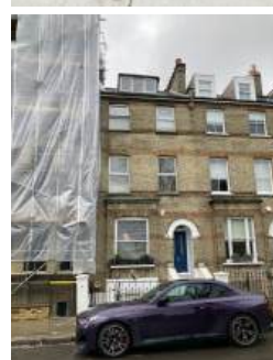
Existing front elevation showing railings and cappings
