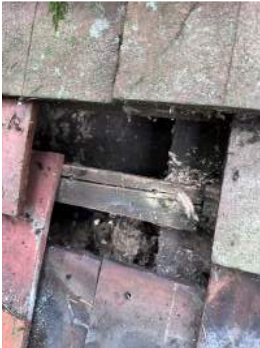
Roof open to void between rafters under tiles
