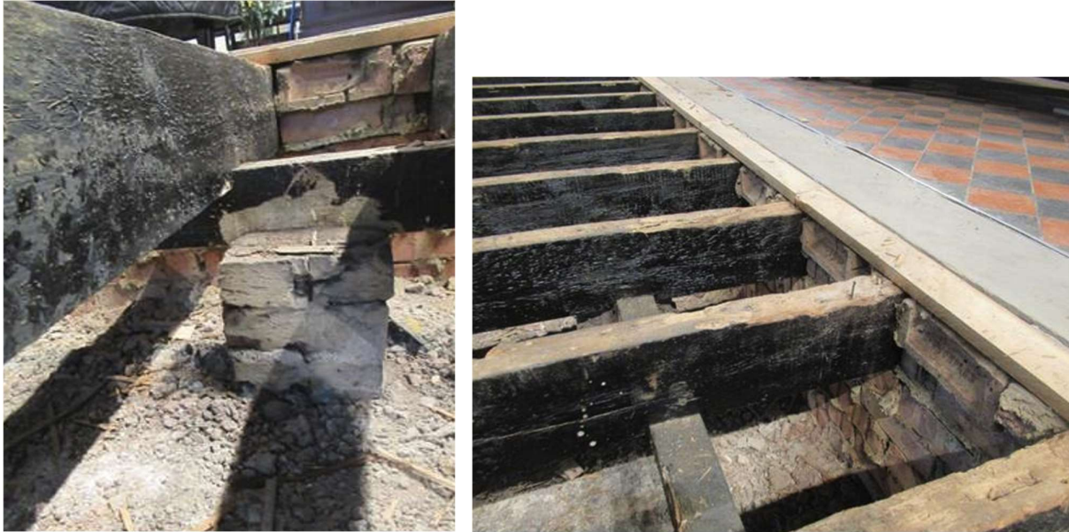
Figure 1 - Photos of existing timber floor structure
