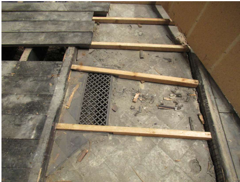
Image 10 – Tiled aisle walkway
