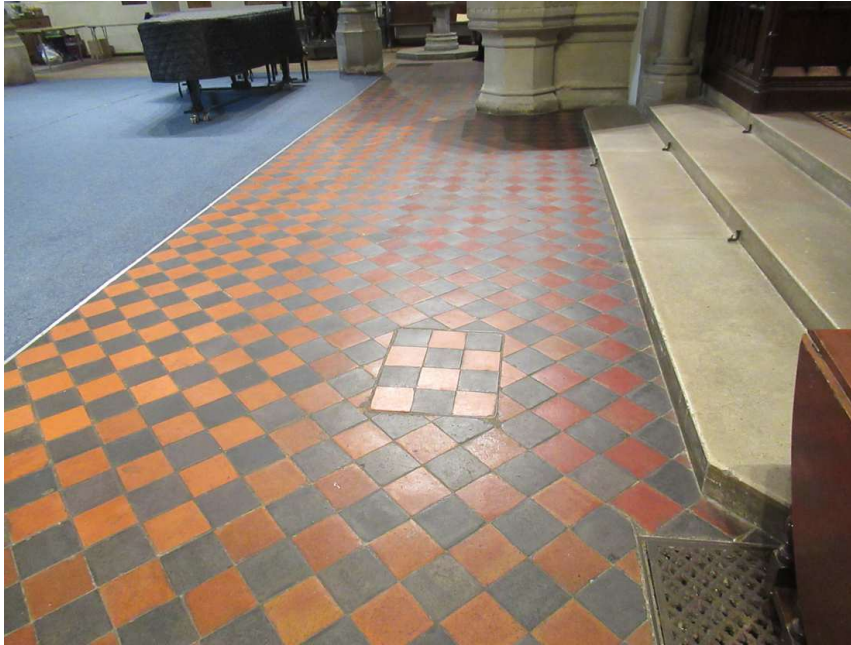
Image 6 – Crossing tiling and chamfered carpet junction
