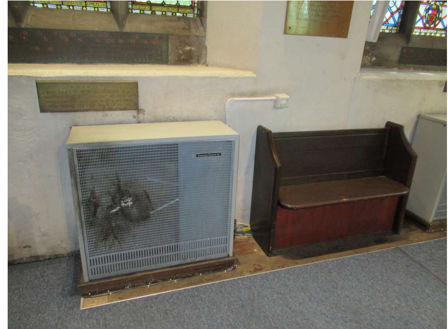
Image 7 – Existing gas heat emitter
