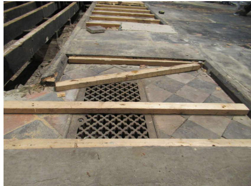
Image 11 – Tiled aisle walkway
