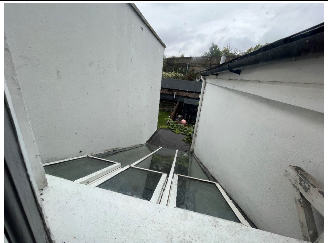
6. Existing rooflight between No.24 and No.25.
