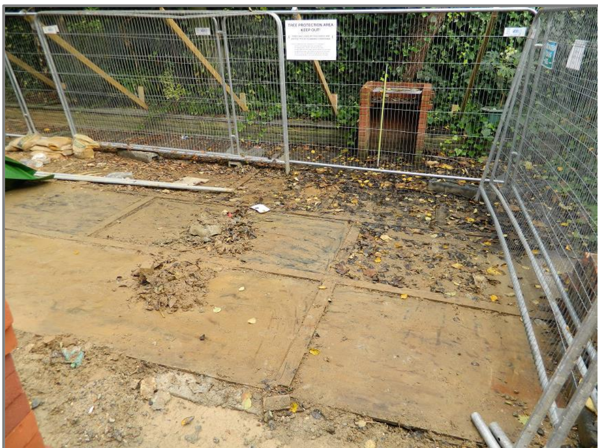
Fig. 7: Illustration of ground protection using plywood over existing paving slabs
