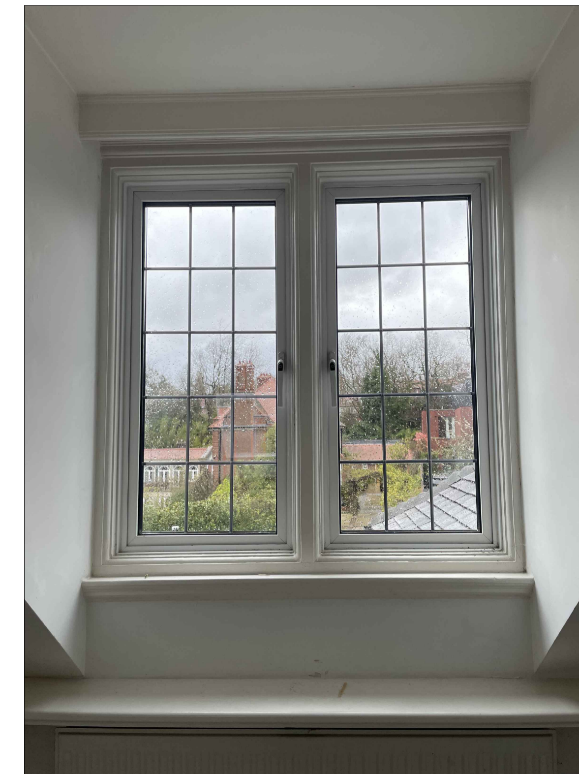
Photo of existing Pvc frame double glazed window with a decorative lead strip overlay on glazing at 2nd floor
