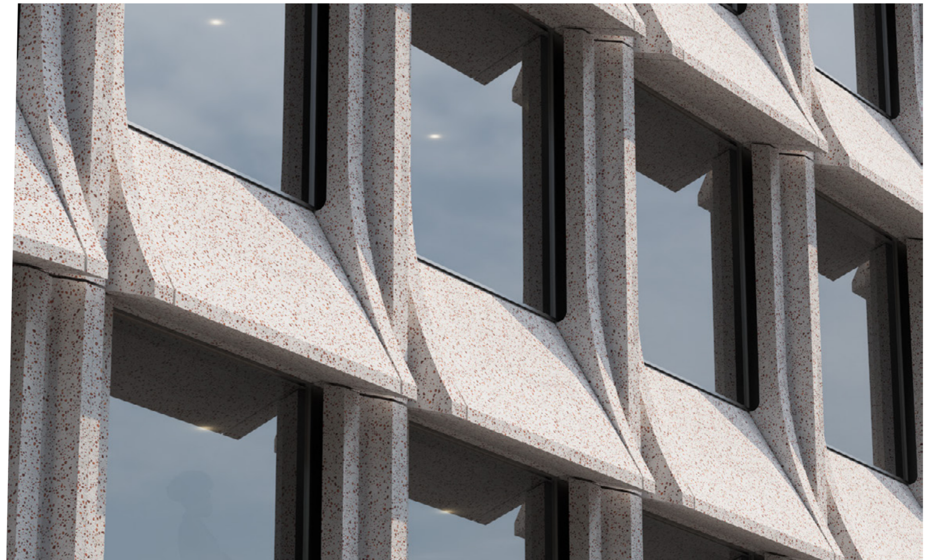
Illustrative View - Exterior view of horizontal and vertical facade cladding shading elements
