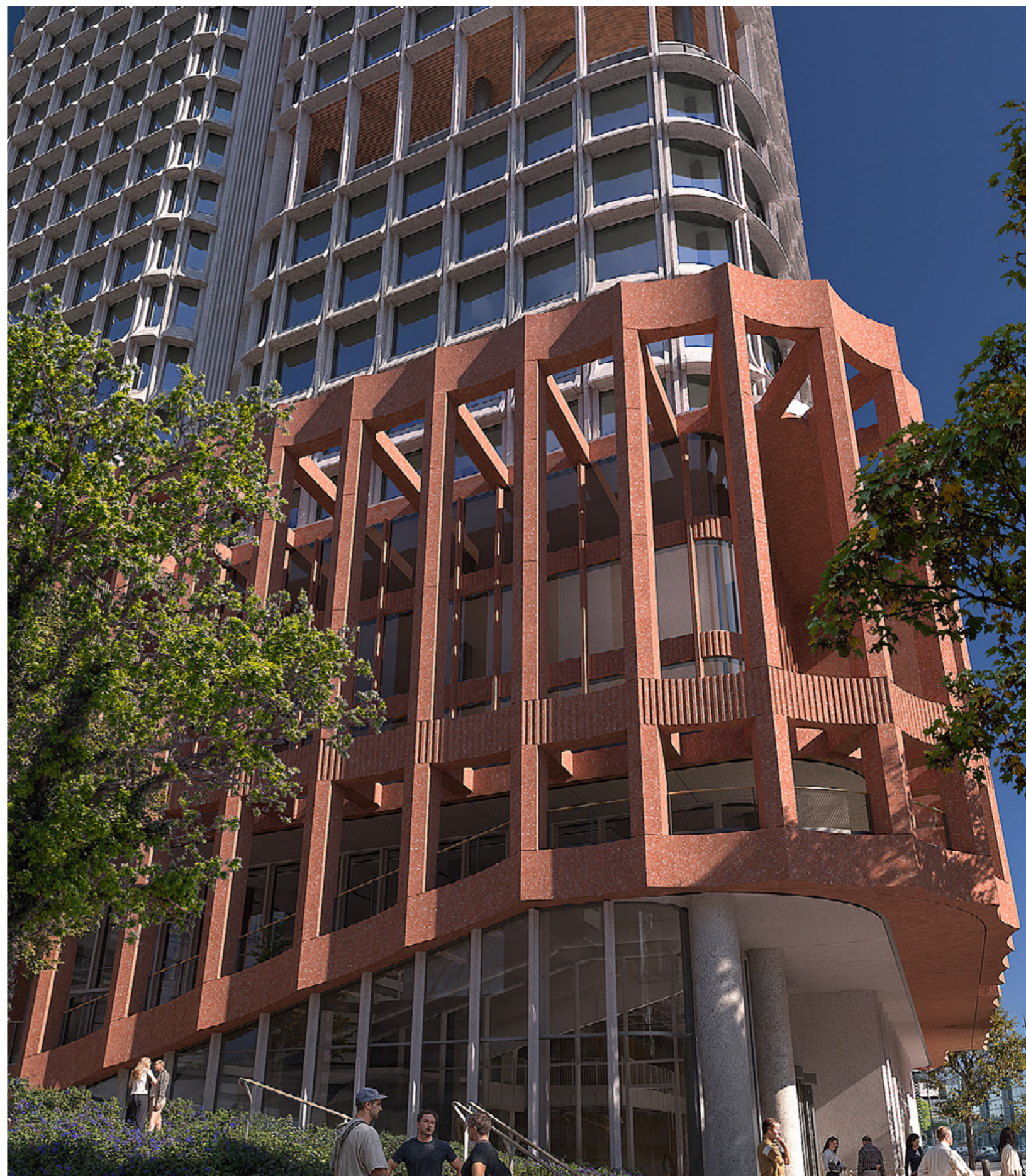
Illustrative View - Looking up at the L11-12 amenity terrace from Regent's Place Plaza
