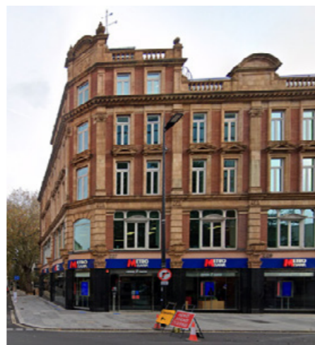
I Filleted Corner at Junction 220-226 Tottenham Court Rd.
