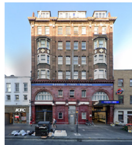
J Colour Change at Lower Levels Goodge Street Station
