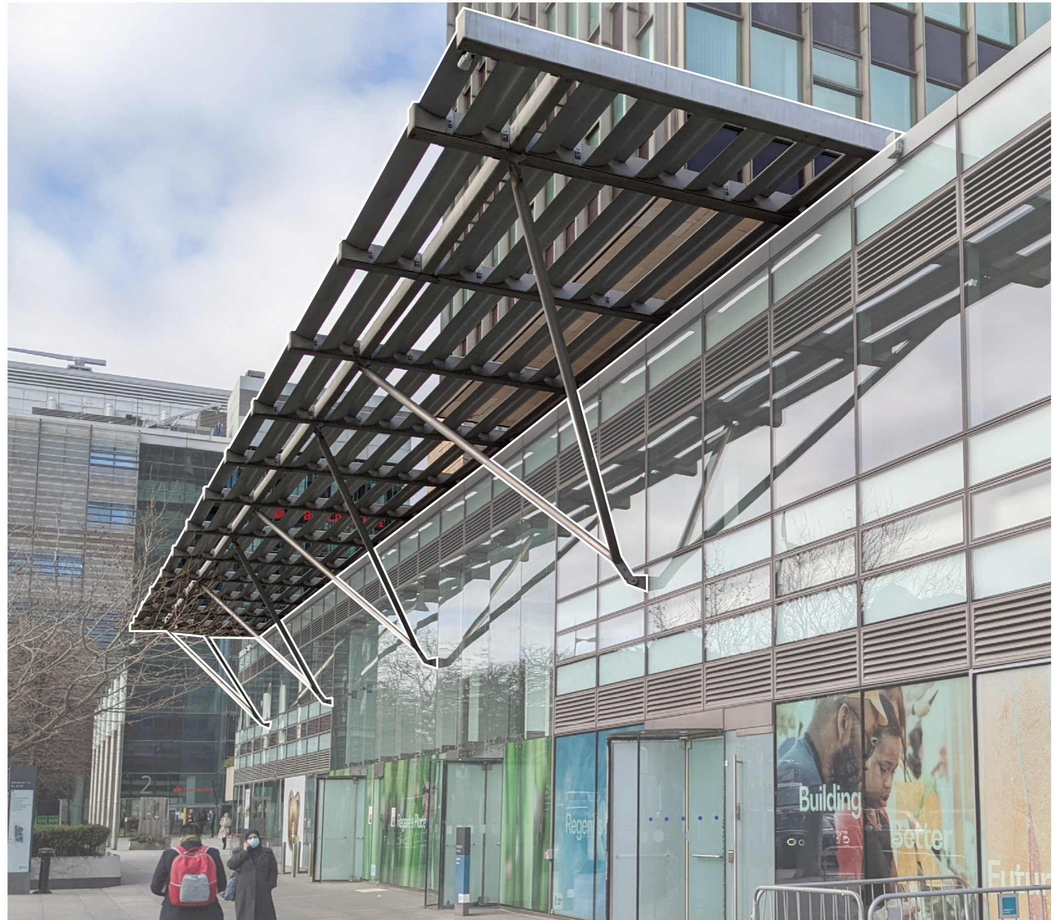
Photograph - Euston Tower wind mitigation canopy, installed early 2000s
