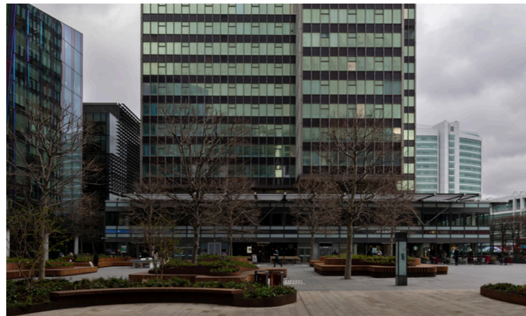
Photograph - Existing Regent's Place Plaza, looking east
