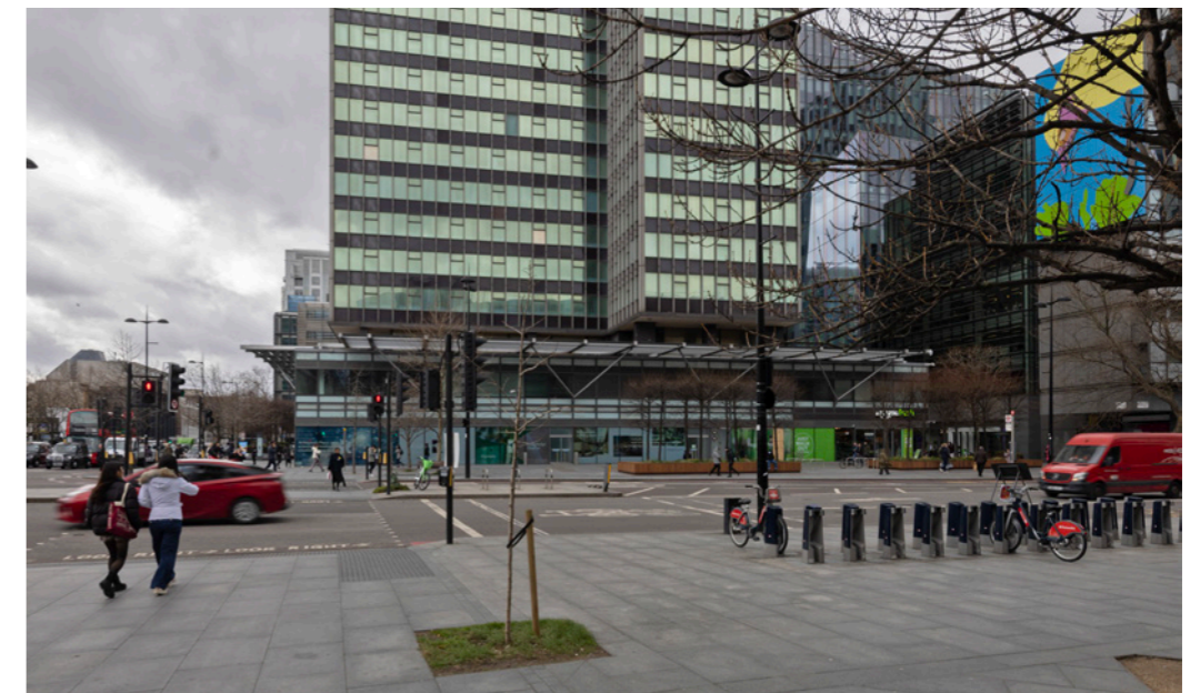
Photograph - Existing Euston Tower ground floor from Hampstead Rd, looking west
