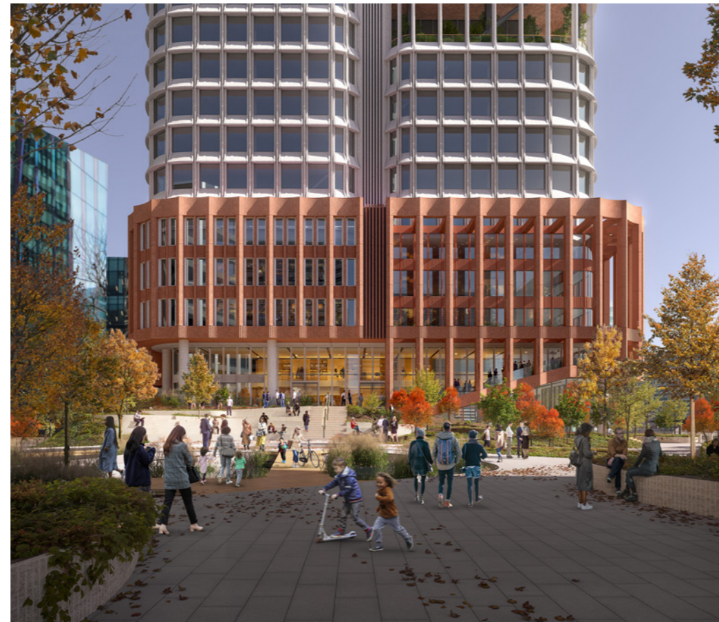
Illustrative View - View to Euston Tower across Regent's Place Plaza
