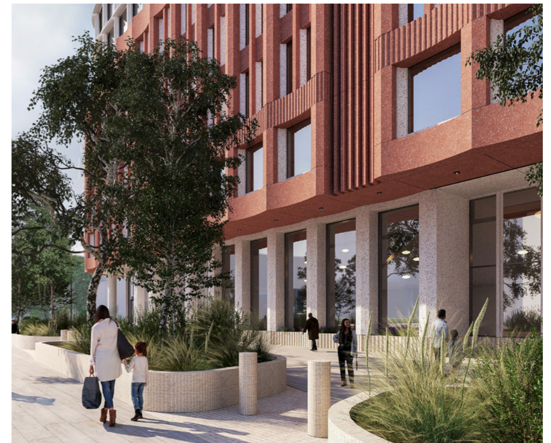
Illustrative View - Looking north along Hampstead Road illustrating interplay between podium facade and planting proposed in public realm
