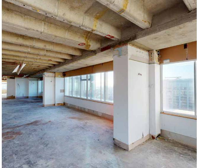
Figure 16.11 Existing ring beam is deeper than the rest of the structural floor system, creating a pinch point for clear floor to ceiling heights once new ceiling services are installed
