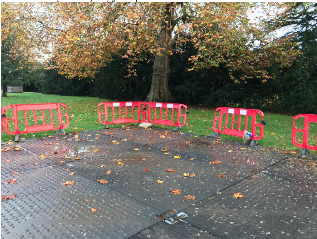
Photo 2. An example of heavy-duty ground protection.
