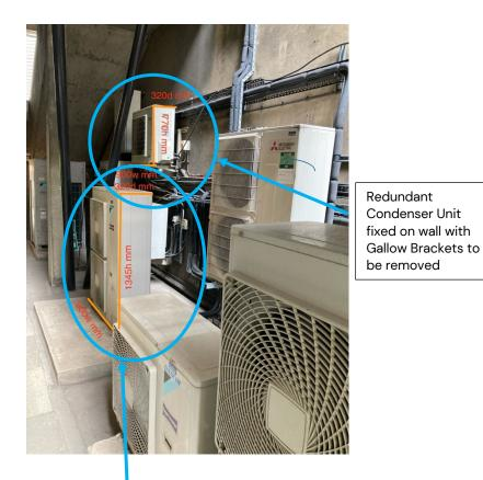
Redundant Condenser Unit to be removed along with associated redundant pipework
