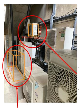
Proposed Condenser Unit to be installed to similar location with new pipework to follow the existing routes
